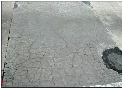
Cracking in Full-Depth Repair
